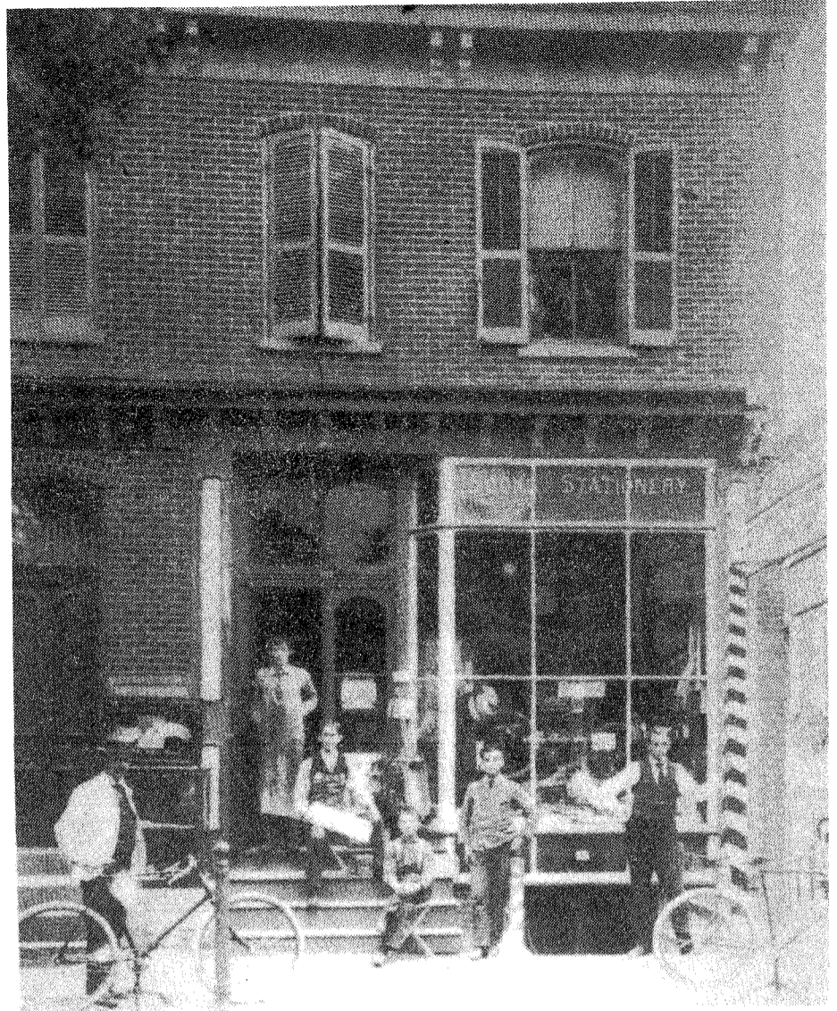
The original office of the old Lititz Express, on East Main Street, now occupied by the Charlotte Heck Antique Jewelry Store. John G. Zook, the publisher, operated a general store
