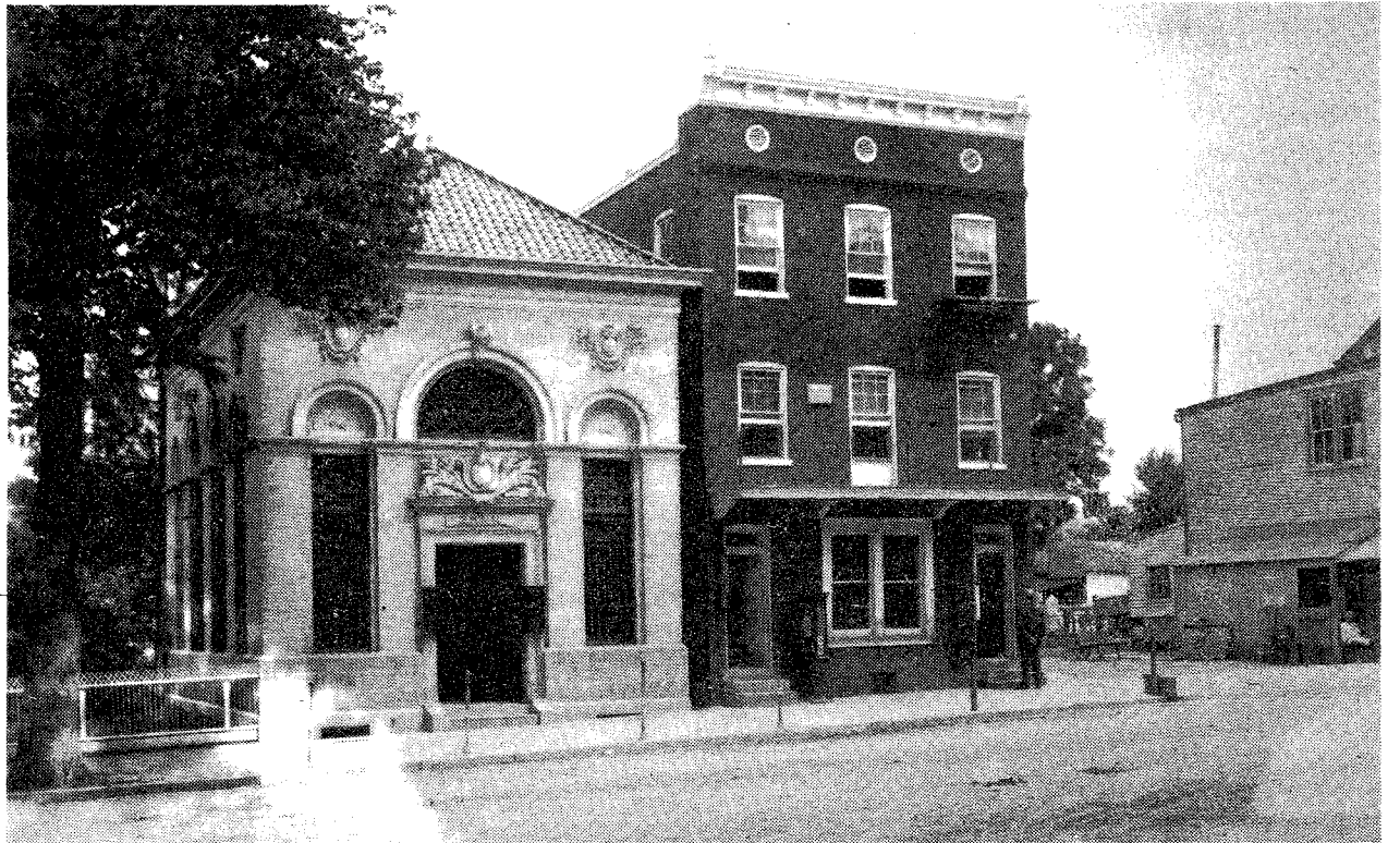
The Lititz Post Office (right), built at the turn of the century, and Lititz Springs National Bank on East Main Street at the Square. A dental and a
