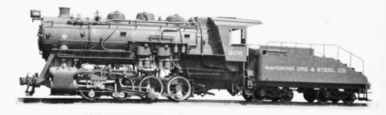
Eight-Coupled (0-8-0 Type) Locomotive for Heavy Switching Service
