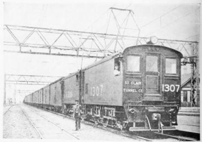
Two of the 66-Ton, 3300-Volt, Single-Phase Baldwin-Westinghouse Motive Power Units Placed in Service on the Grand Trunk Railway in 1908.
