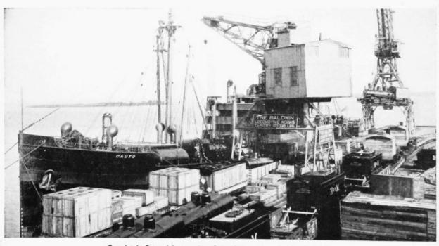
Completely Erected Locomotives Being Shipped from Wharf No. 251
