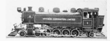
Eight-Coupled 4-8-2 Type Side Tank Locomotive for Freight Service
