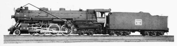
Modern High-speed Passenger Locomotive Equipped with the Elesco Type "E" Superheater and Elesco Feed Water Heater.
