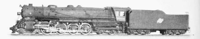
4-8-4 Type Locomotive for Passenger and Freight Service Built for the Chicago & North Western Railway Cylinders 27 in. x 32 in. Drivers, diam. 76 in. Weight, total engine 498,000 lb.
