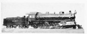
Santa Fe (2-10-2) Type Locomotive with Tandem Compound Cylinders Built for the Archison, Topeka & Santa Fe Railway, 1903 Cylinders 19 in. and 32 in. x 32 in. Drivers, diam. 57 in. Weight, total engine 287,240 lb.
