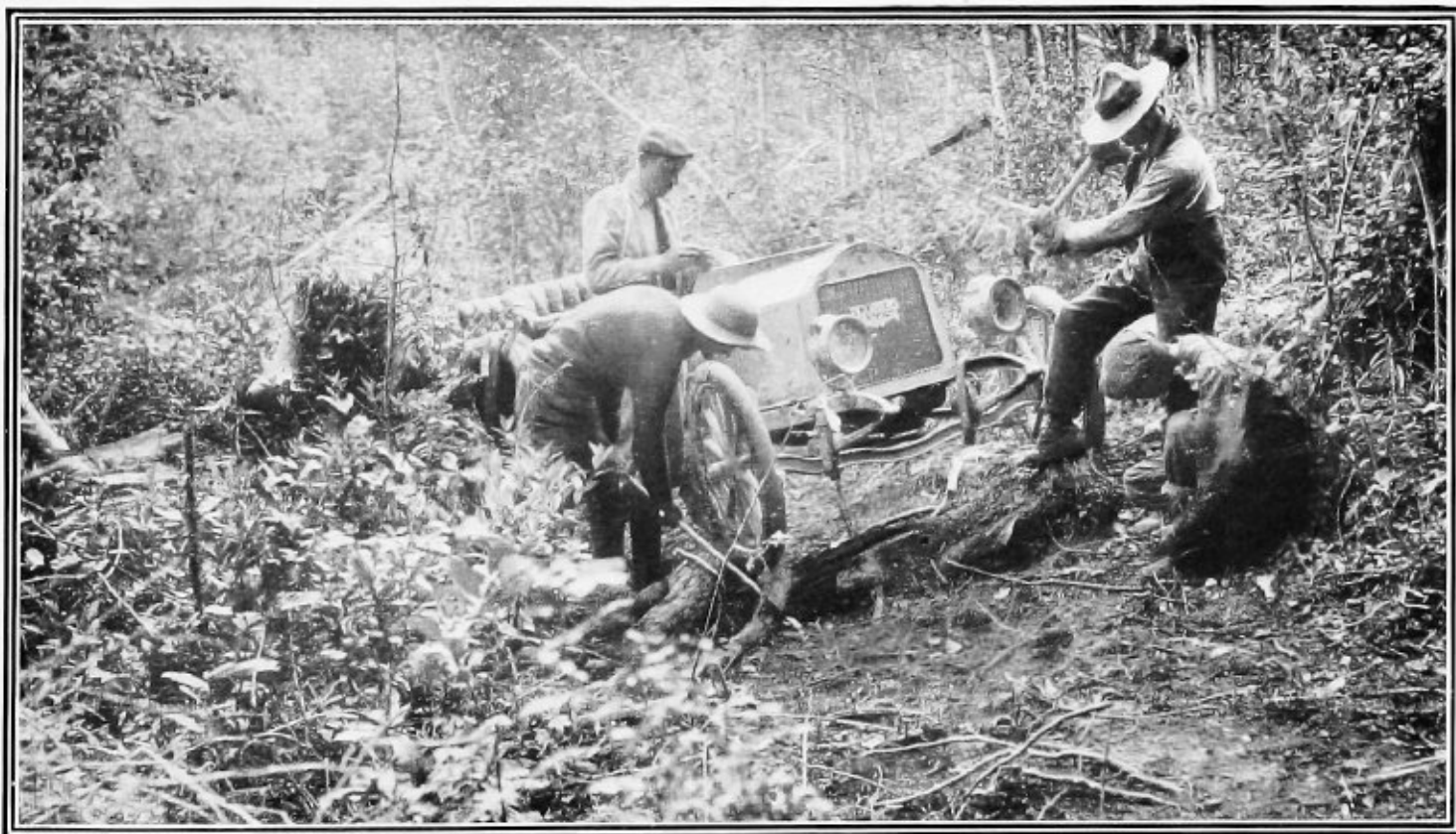
Clearing the way for the "First to Hazelton" Flanders "20." Often it was necessary to fell trees and dig out stumps to give the car room to pass
