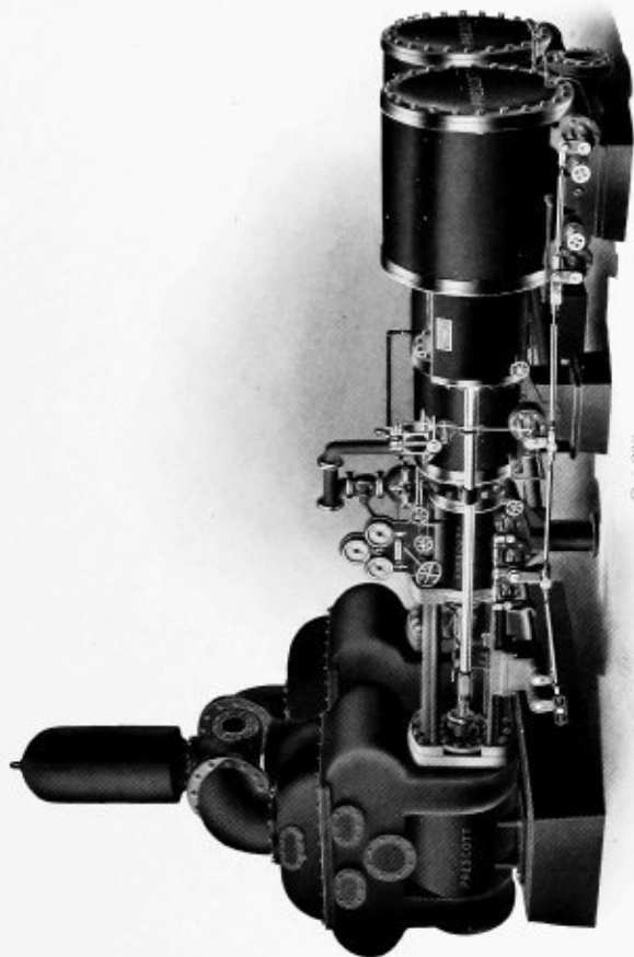
Prescott Triple Expansion Low Service Pumping Engine Separate Water Cylinders
