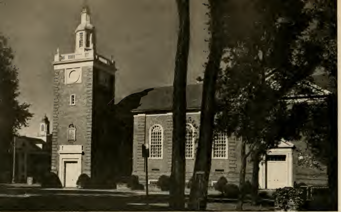
A new view of a familiar building on Lycoming College campus. Clarke Memorial Chapel.
