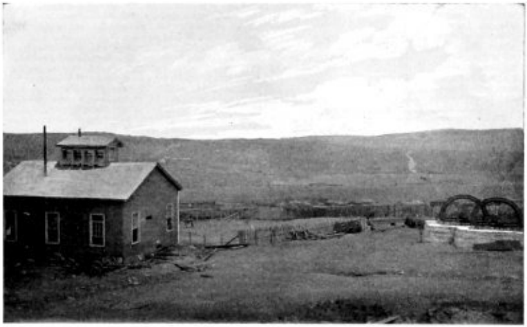
FIG. 8.—VIEW OF SURFACE ARRANGEMENTS FOR HOISTING ON INSIDE SLOPE. ROPES PASS OVER THE SHEAVES AND DOWN BORE-HOLES.
