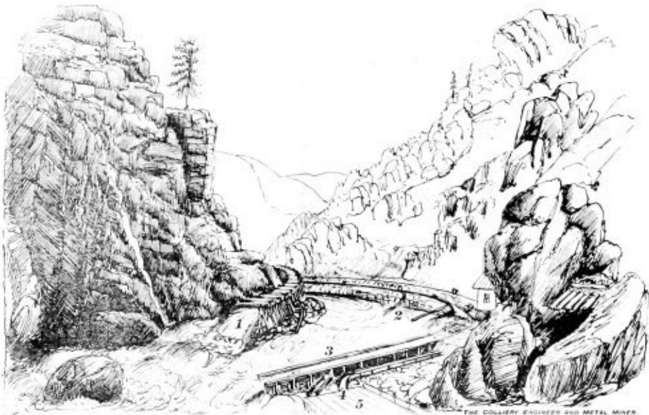
SLUICES AND FLUME AT THE STONE DAM.
