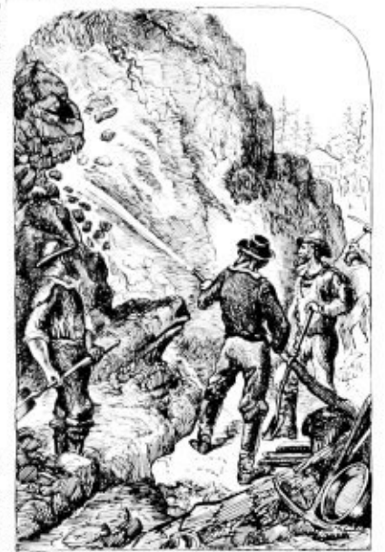
FIG. 4.—THE FIRST ATTEMPT AT HYDRAULIC MINING.
