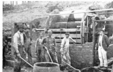
CAPPELL FAN IN COURSE OF ERECTION AT MOON RUN, PA.
