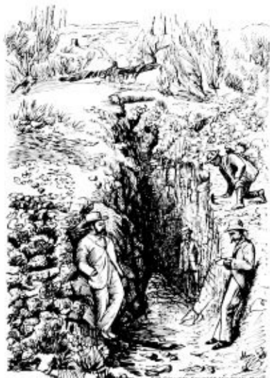
QUARRY IN MANGANESE SHOWING 25 FT. FACE THICKNESS OF SOLID MANGANESE.
