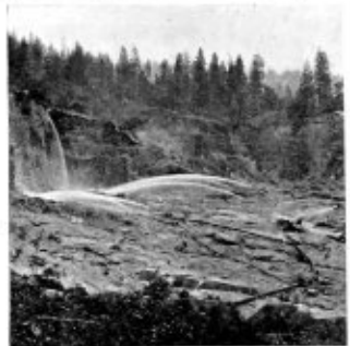
FIG. 5.—CAVING PLACER BANKS IN CALIFORNIA.
