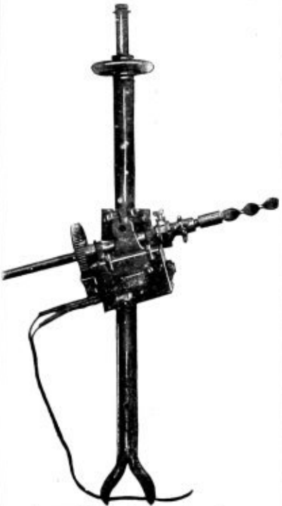
JEFFREY IMPROVED ELECTRIC COAL DRILL.
