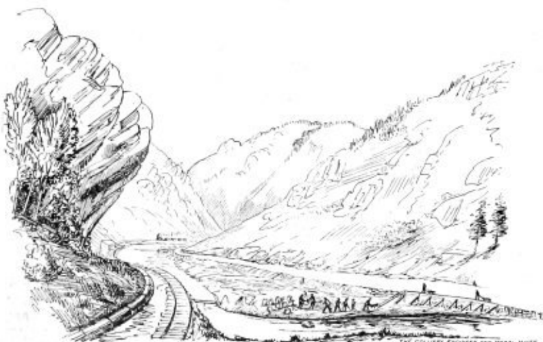
FIG. 3.—MAKING EMBANKMENT OF FLUME, SHOWING PIPE AND FLUME.
