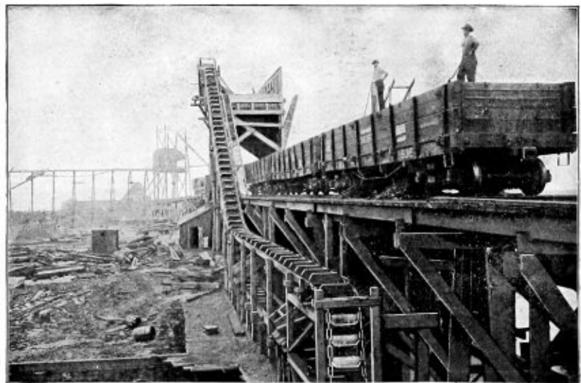
THE JEFFREY CONVEYING MACHINERY FOR COAL VESSELS.
