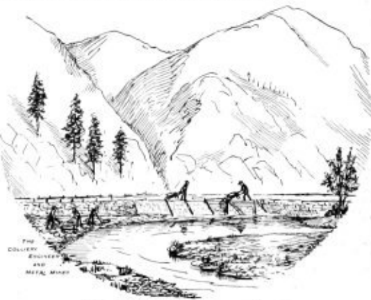
FIG. 2.—MAKING EMBANKMENT OF FLUME.
