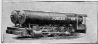
Compressed Air, Main Entry
