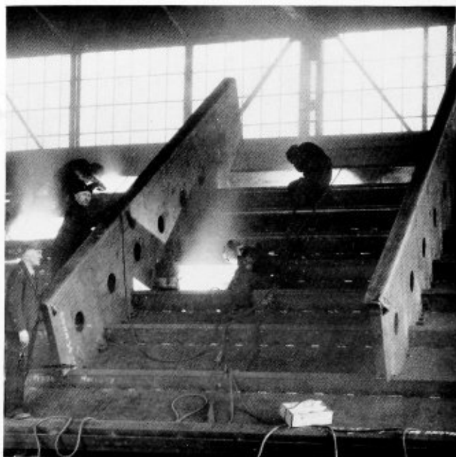
Fabrication project in which new fillet electrodes were employed
