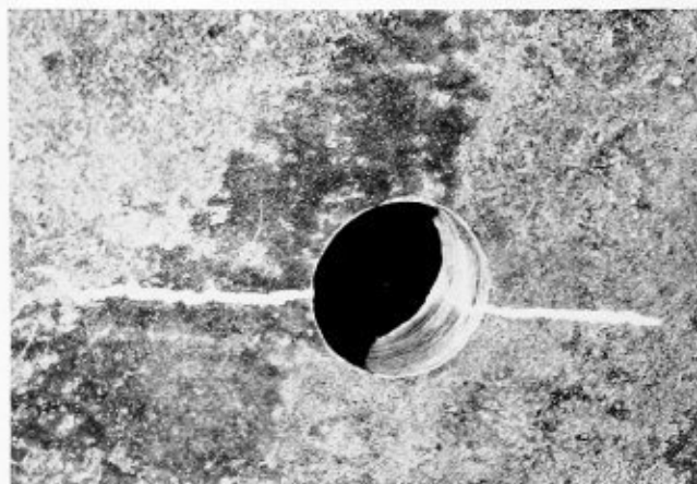
Fig. 3.—Crack in 1\frac{1}{16} -inch shell plate
