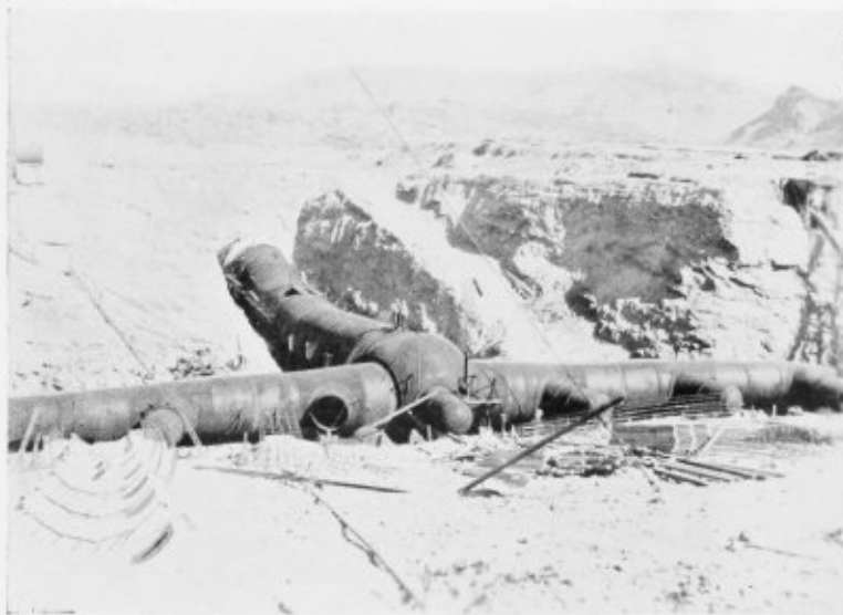
Giant welded inlet manifold for Colorado River Aqueduct
