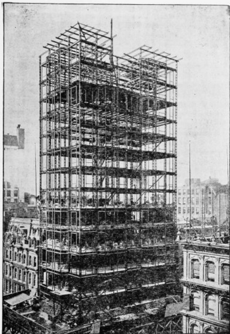
Reliance Building, during Construction. Aug. 1, 1894.
