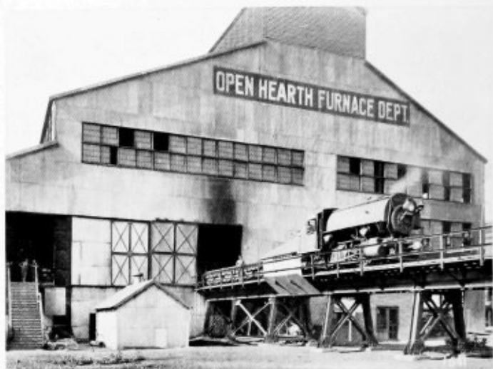
"Locomotive drawing train of charging pans through the Open Hearth Department."
