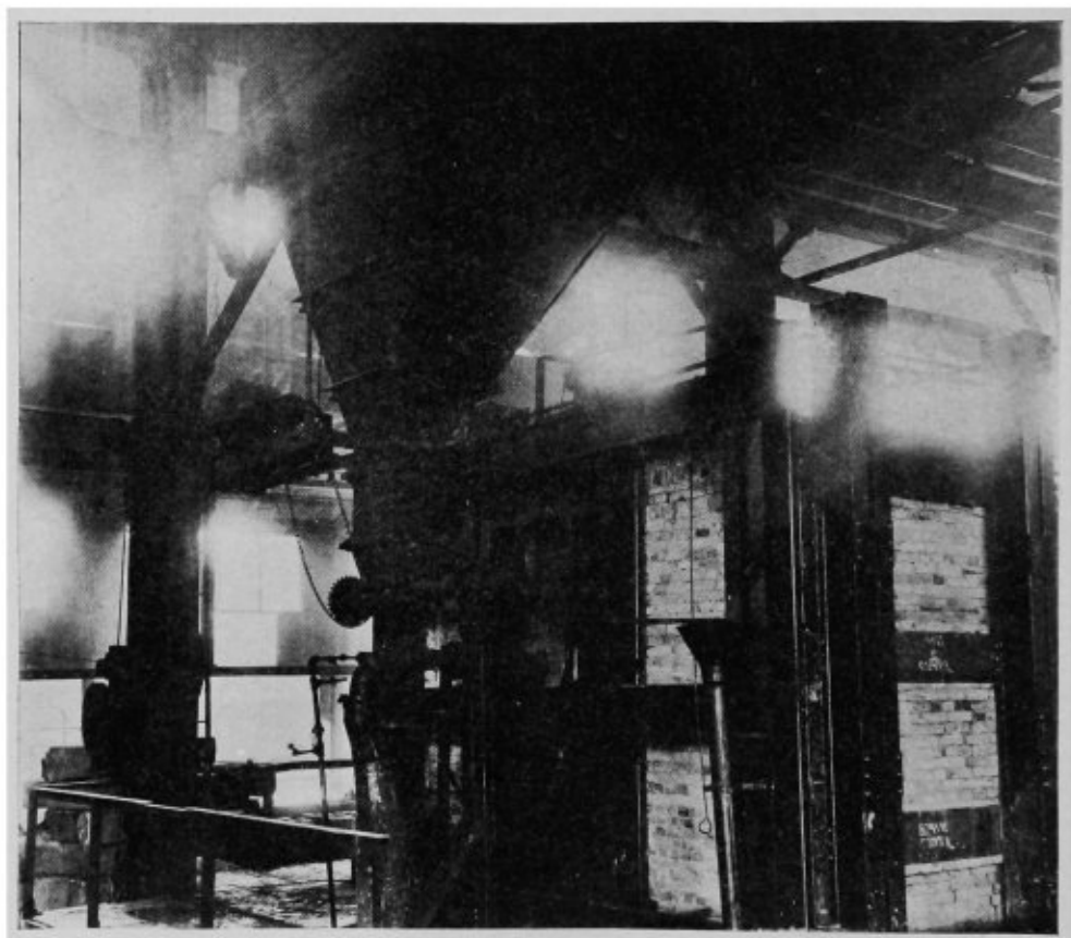
Bin, feeder, and burner used on a 50-ton Open Hearth Furnace, using pulverized coal.
