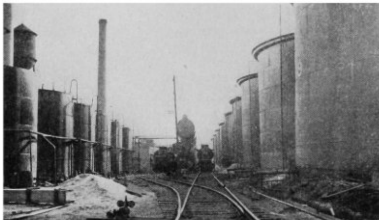
Crude Tar Storage Tanks
