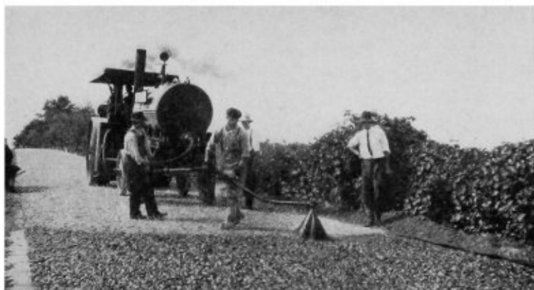
Spreading Tarvia on Wearing Course
