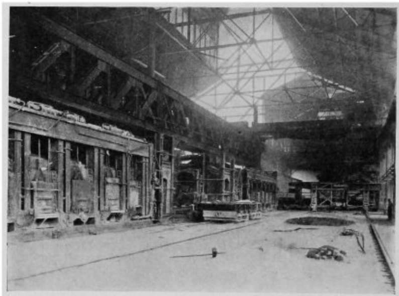
FIG. 5—Charging Side of Furnaces.
