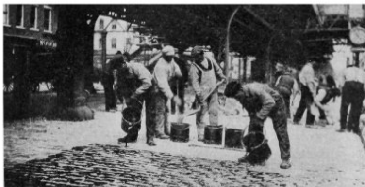
Mixing and Spreading Pitch and Sand Filler on Belgian Block Pavements
