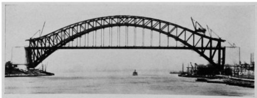
Entire floor in place. Back stays and one arch traveler dismantled.
