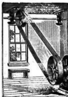
Baker Pressure Blower Driven by Belt.
