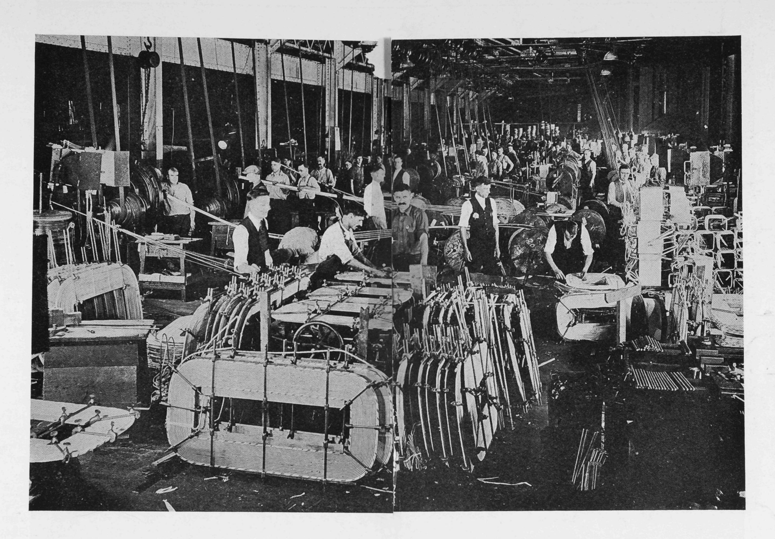
Section of the coil-winding department where coils large Westinghouse turbo-generators are wound C
